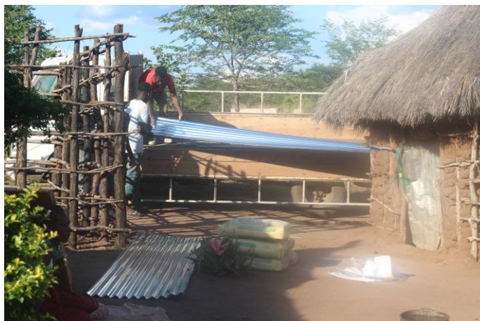
ECCT Drivers deliver iron sheets on site.
