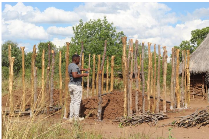
Senior Social Worker, Gift, inspecting the project's progress.
